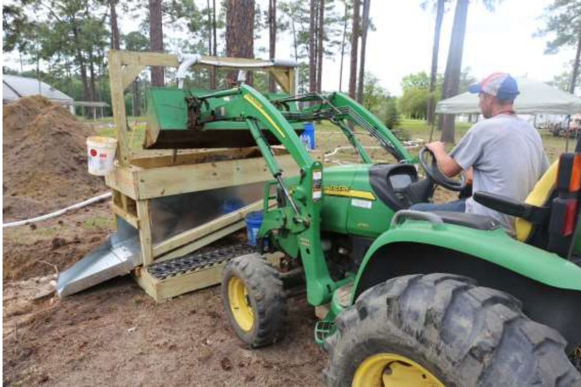
Figure 47. Soil is placed into screens for shifting.
