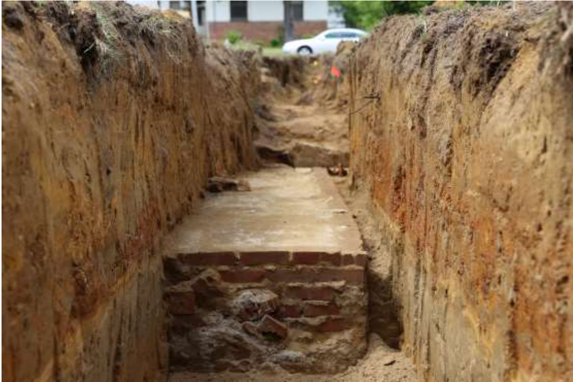
Figure 51. Trench 3, facing north. Buried brick structure is the top of an underground tunnel.
