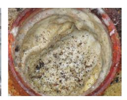
One of the worst things that can happen to a home or business is discovering a sewage overflow due to plumbing problems. More often than not, when those overflows are investigated the cause is clear — fats, oils and grease (FOG) have clogged the pipes and prevented it from performing its duty.
