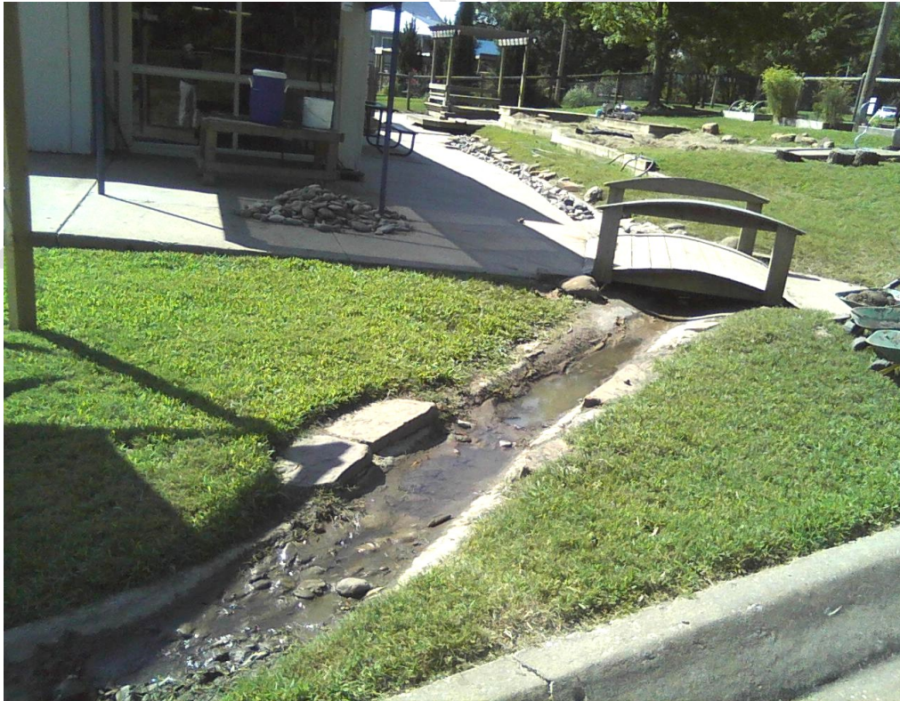
Picture 4. Open Drainage Channel Conveyance; North End of Building #1.
