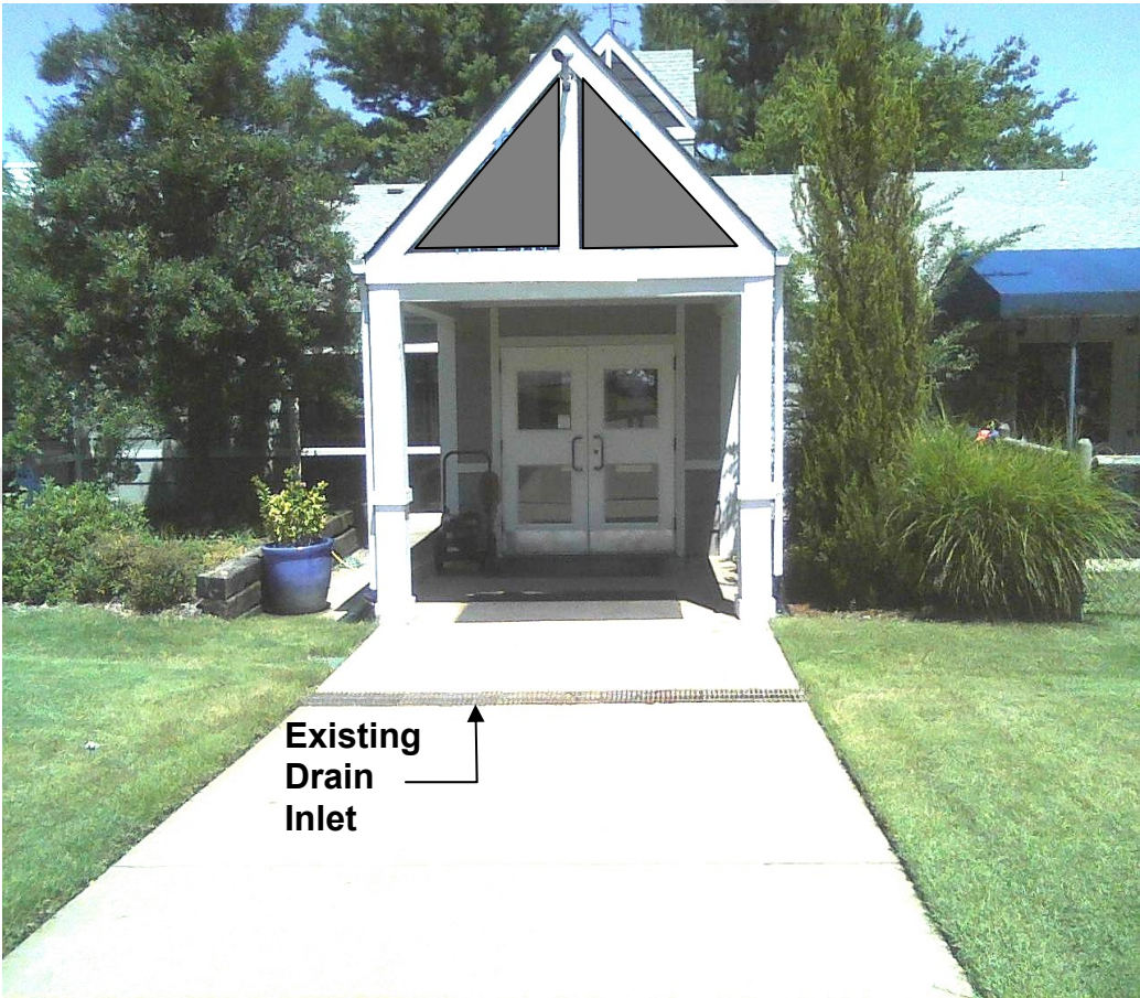
Picture 1. Entrance to Building 1; Existing Interception Grate. Looking NE
