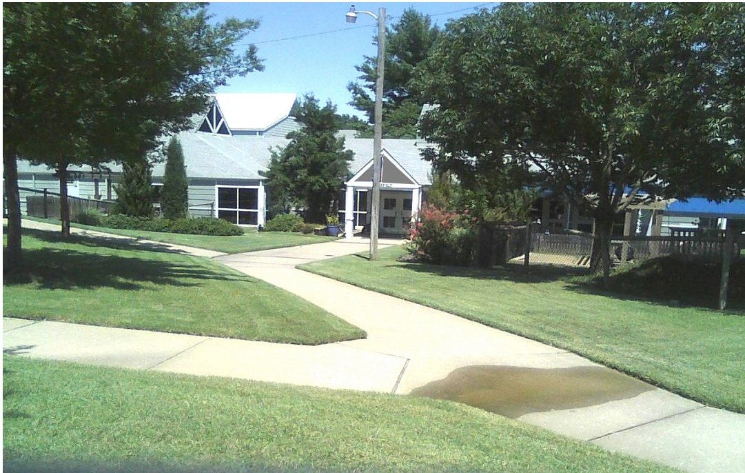
Picture 2. Entrance to Building # 1, Looking Northeast
