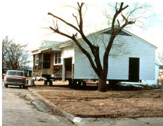
Moving a home out of the floodplain is sometimes the only way to protect it from flooding
