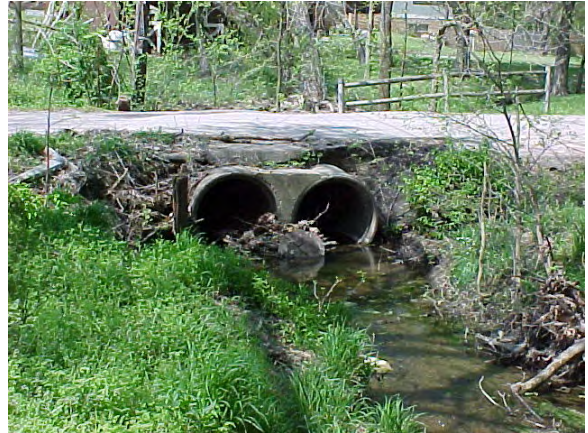
Culverts like this one can constrict flow and cause backwater flooding
