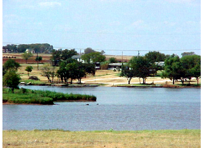
Reservoirs provide storage of rainwater without the hazards of maintaining a dam
