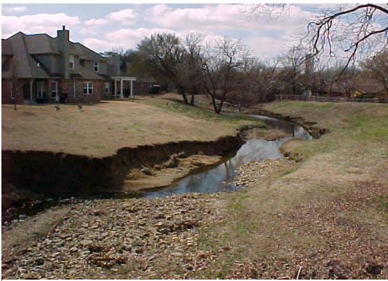
Lack of vegetation along drainage channels promotes erosion
