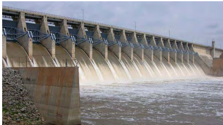
A release of 40,000 cubic feet per second (cfs) from Keystone Dam, upstream of the City of Tulsa
