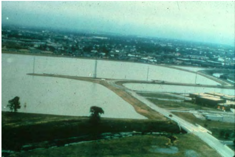
Stormwater Detention Ponds manage the increased runoff from new developments, temporarily store flood waters, and can be used for community parks, recreation, and open-space
