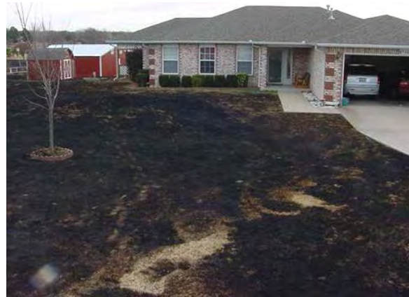
A home in the WUI surrounded by a “defensible” zone that helped protect it from damage during a wildfire outbreak
