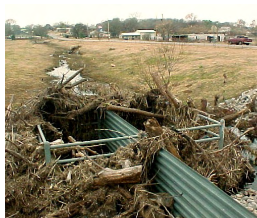
Drainageways are inspected regularly for blockage from debris
