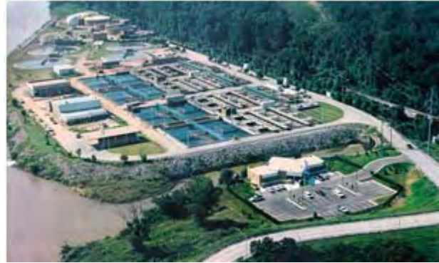
Southside Wastewater Treatment Plant
