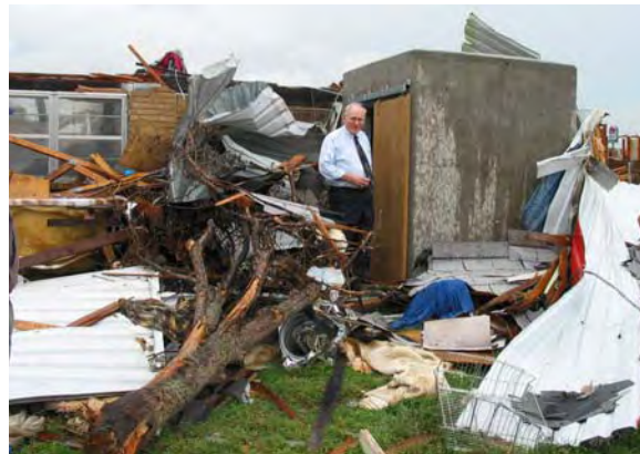
Dr. Ernst Kiesling, Civil Engineering Professor at Texas Tech University inspects a safe room in the aftermath of the May 8, 2003 tornadoes in Moore, Oklahoma.
