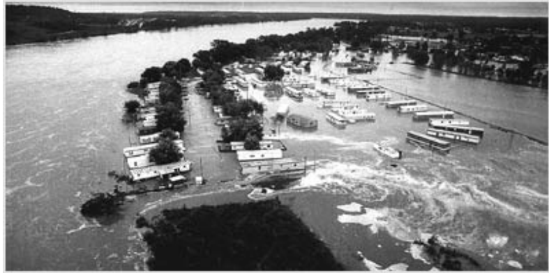
A Sand Springs levee gives way during 1986 flood on Arkansas River
