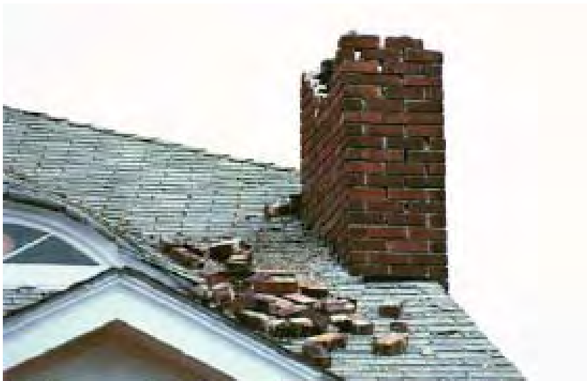
Although located in the relatively quiet Central Plains Province, nearness to the New Madrid, Missouri, fault exposes some Oklahoma communities to VI intensity tremors
