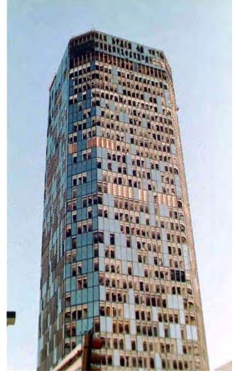
The glass-clad Bank One Tower, Fort Worth TX, following the March 2000 storms. (Photo by Doug Smith, AAWE)
