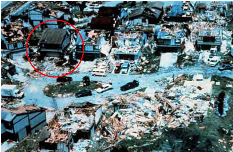
Illustrating the dangers of unreinforced garage doors, in all but the house at upper left, these doors have been breached, leading to substantial roof damage – in some cases, completely removing a second floor. But in the home with an intact garage door, the roof is almost entirely undamaged.
