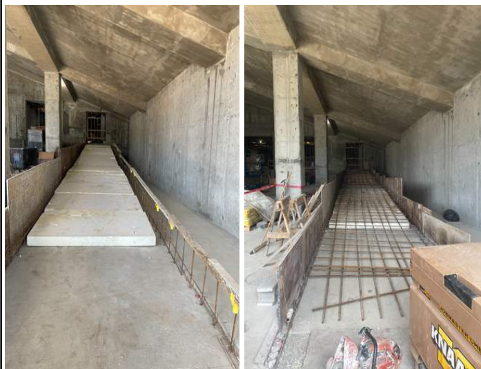
Loading dock ramp is currently in progress.
