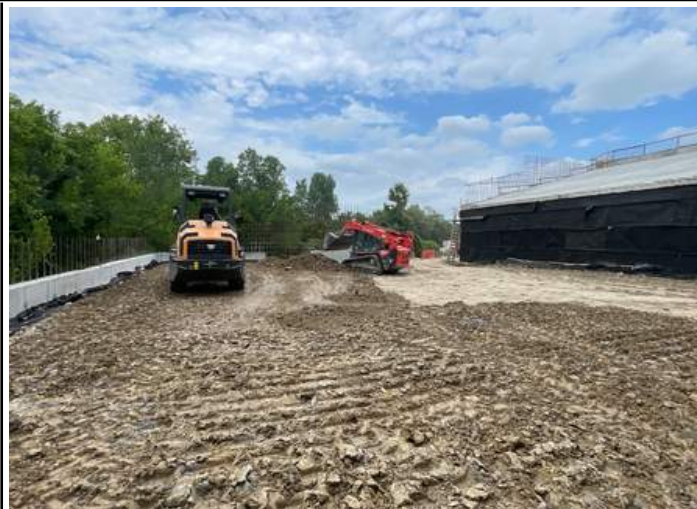
Backfill of the amphitheater is currently in progress.
