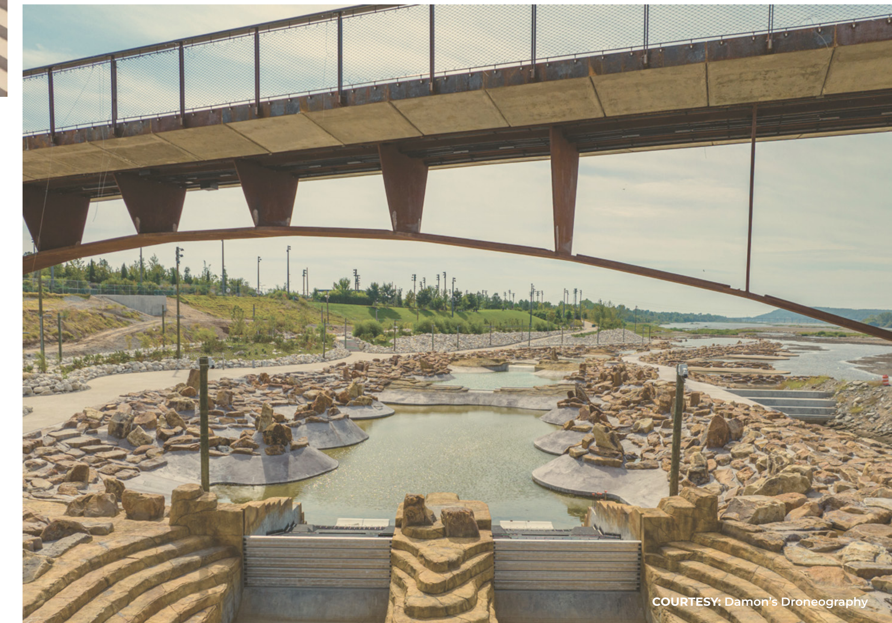
CONTINUED PROGRESS: ZINK DAM & PEDESTRIAN BRIDGE
