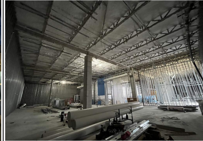
L2 gallery framing and rough-in in progress.
