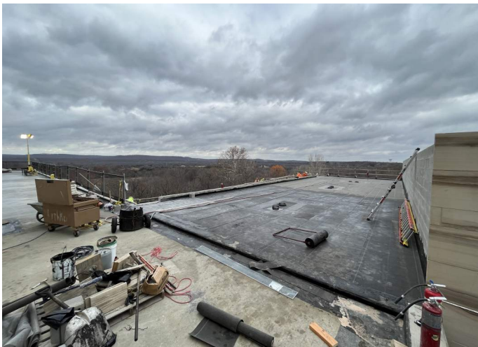
L1 Amphitheater patio waterproofing on-going.
