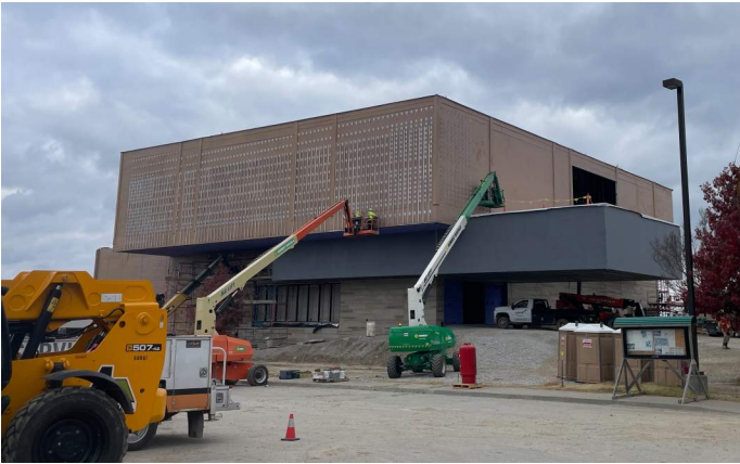
Main building view -- Metal panel substructure in progress --
