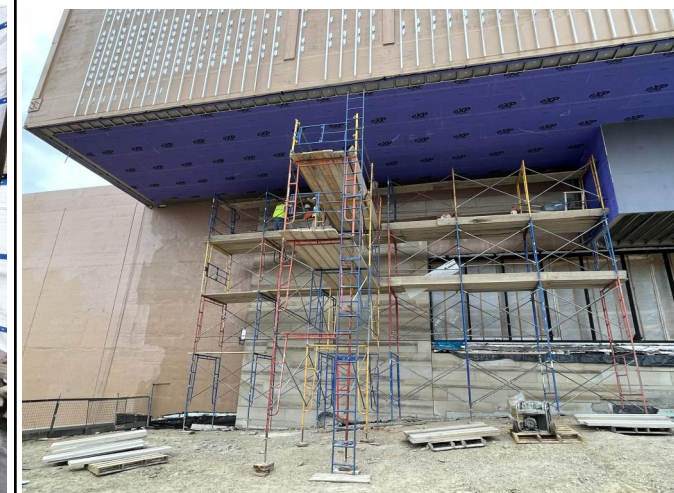
Stone is in progress on the south facade.
