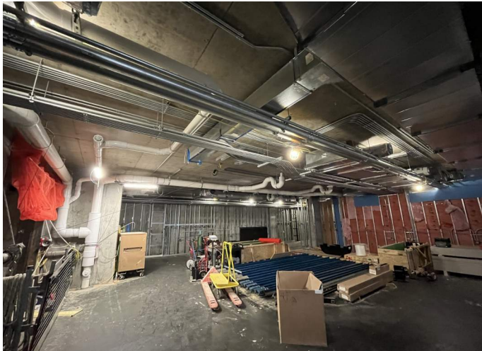
LL2 gallery framing and rough-in in progress
