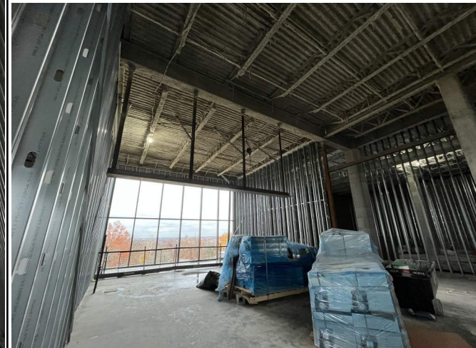
L2 gallery framing and rough-in in progress.
