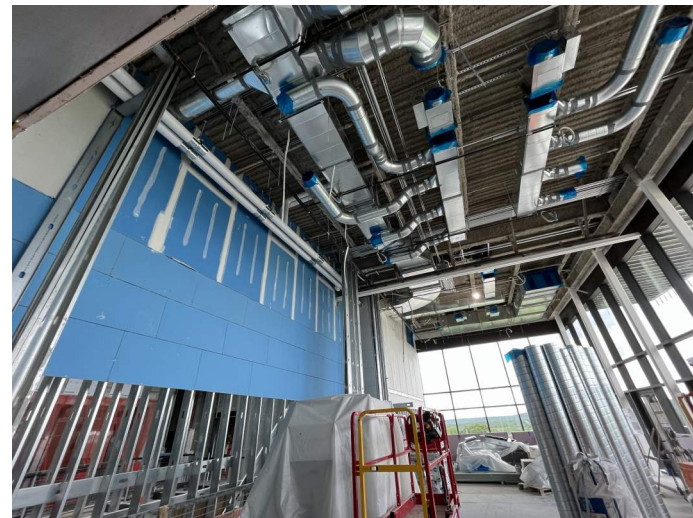
Special events L2 overhead rough-in and drywall are in progress.
