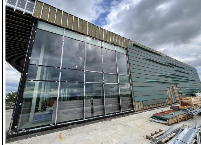
West metal panel soffit is in progress.
