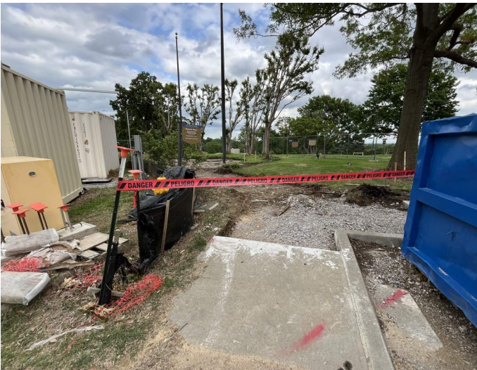
East site sidewalk demolition is in progress.
