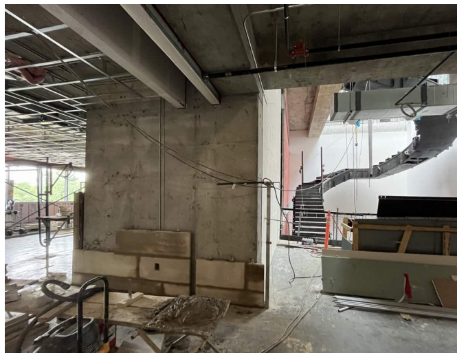
Interior stone veneer progress at main entry lobby continues.
