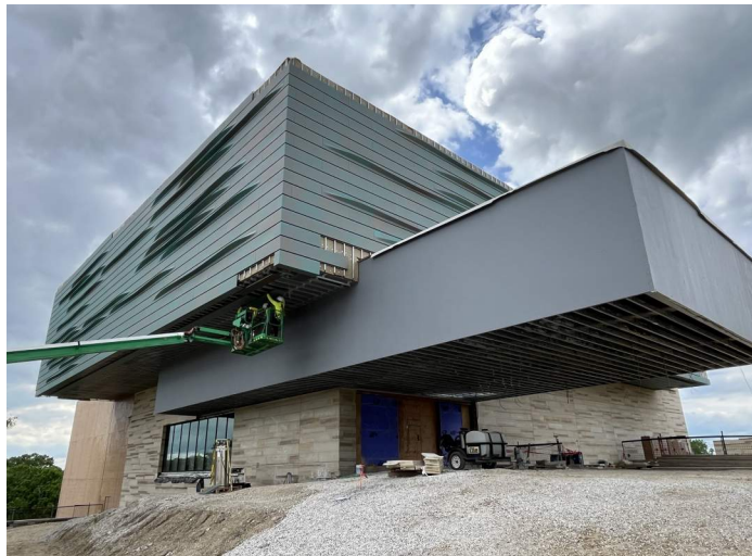
South metal panel facade & soffit is in progress.
