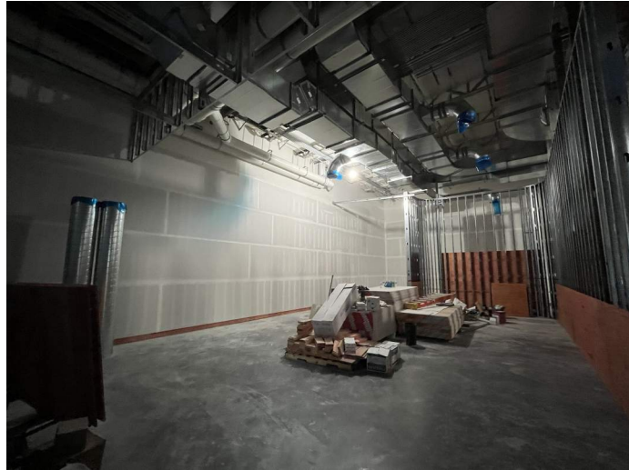
L2 drywall and plywood in galleries are in progress.
