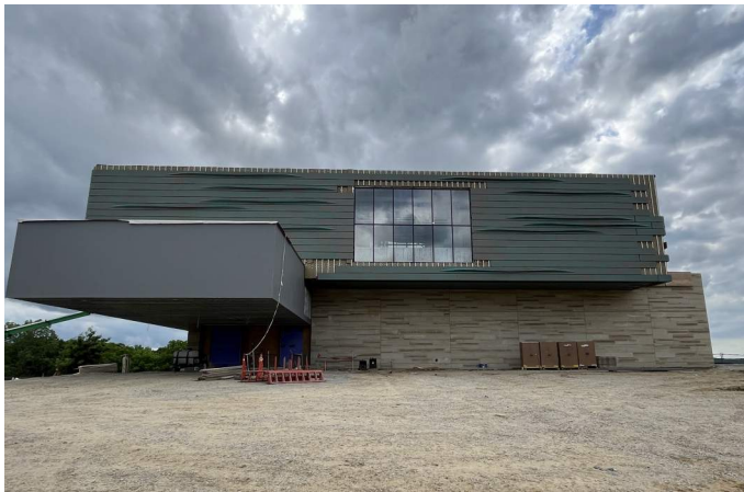
Main building view -- Metal panel installation in progress --
