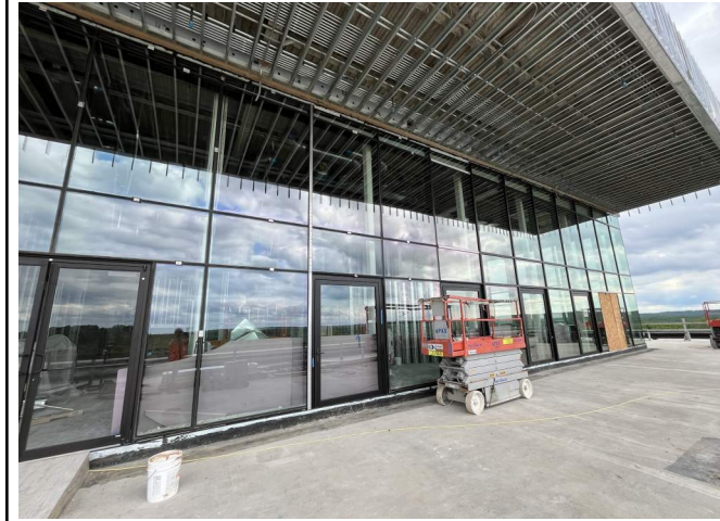
Pivot doors at L2 terrace are installed.
