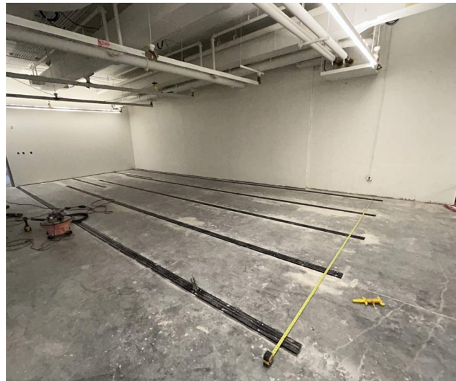
LL3 high density shelving recessed floor tracks install is in progress.
