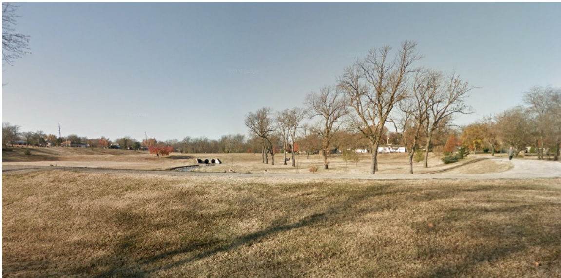
Jones Creek stormwater detention facility, looking upstream from E. 14 th St. and S. 79 th E. Ave.
