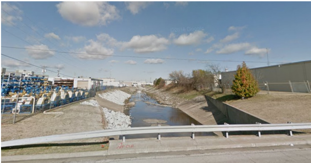
Looking north on Mingo Creek towards RLA #9 from the E. 55 th Pl. bridge.
