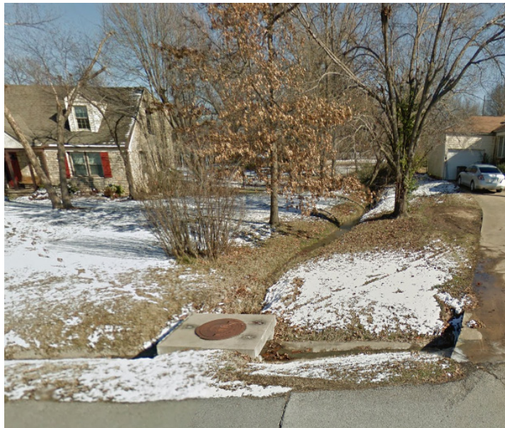
This drainage cut between properties follows the original ELB.3A stream bed to the storm sewer on S. Darlington Ave.
