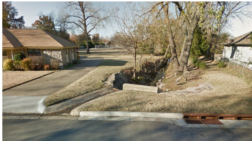
Little Joe Creek channel, looking north—downstream—from E. 58 th St.
