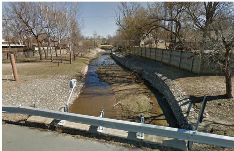
Looking east (upstream) on Fred Creek from Harvard Ave. bridge.
