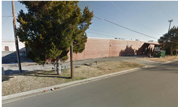
Property 1 in RLA #36 backs onto S. Maplewood Ave. and acts as a barrier to overland flow runoff coming down E. 21 st Pl. and E. 22 nd St. from the high ground along S. Fulton Pl.
