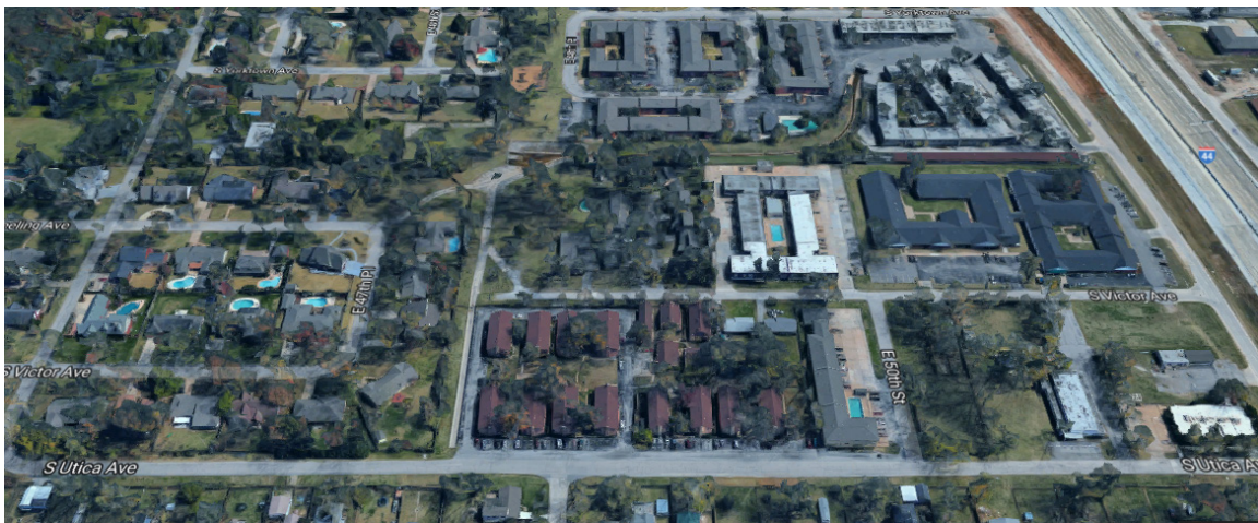
Looking out over South Bolewood and RLA #51 from the west, with E. 47 th on the left of the picture and I-44 on the right.
